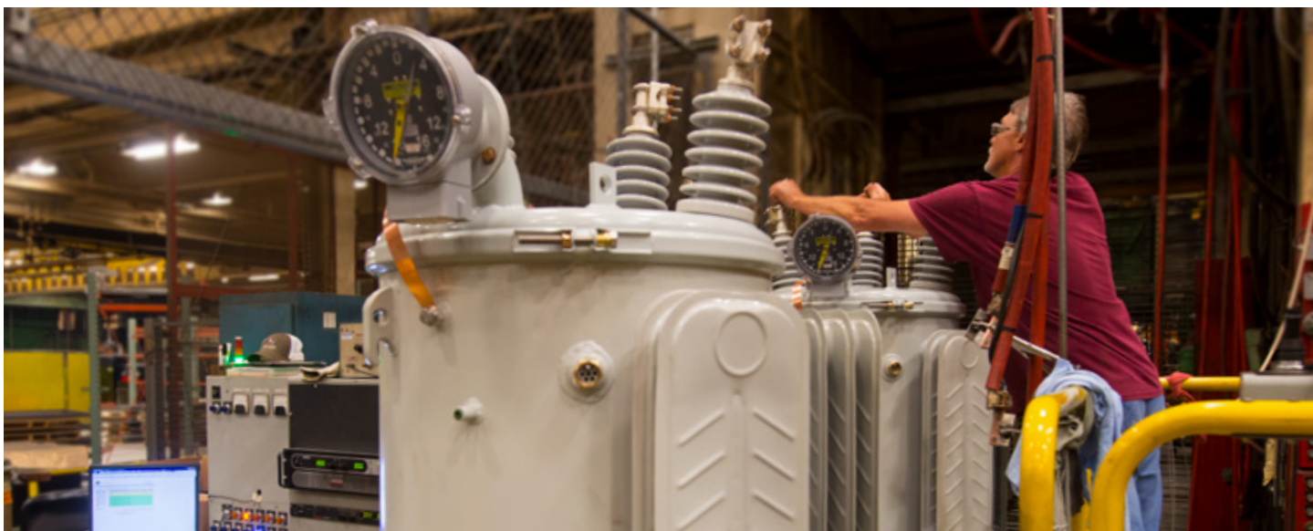
Complete electrical testing
