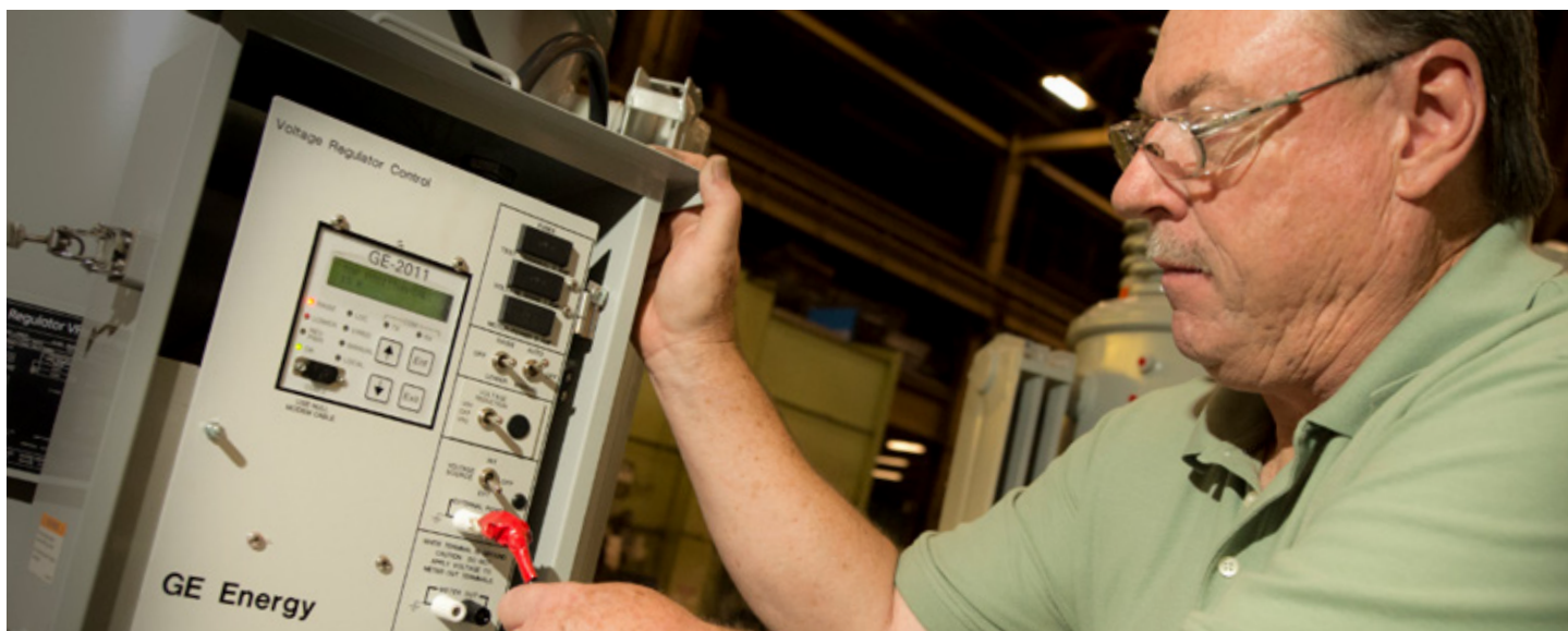
Controls programming and testing
