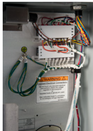
Terminal, Terminal Covers, and Independent Ground Plate Back Plane
